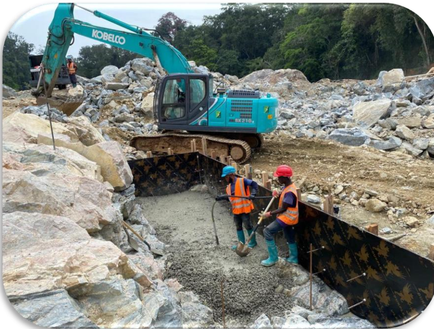
Figure 5: Kaiha II decommissioning of the dam site
